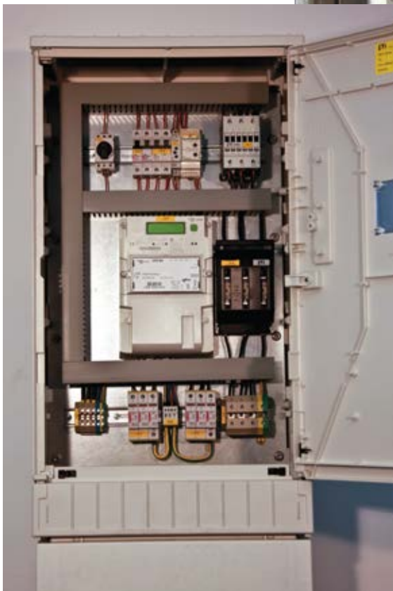
Meter distribution cabinet
